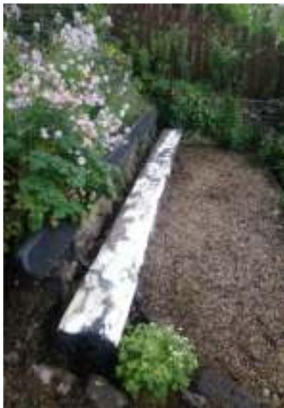
Once back to mostly bare wood, I applied the wood hardener to the worst areas of spongy timber and then filled holes, cracks and missing areas with filler. Finally I applied two coats of black paint.
